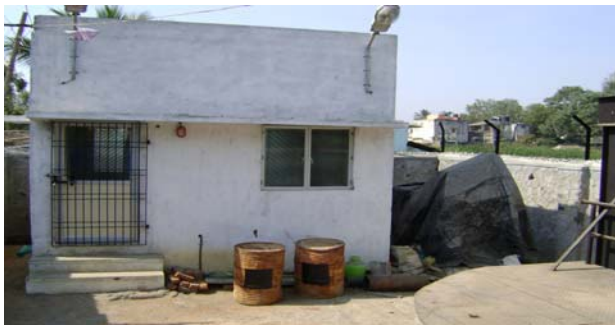
Arulmurugan Lifting Station
