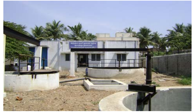
Indira Nagar Pumping Station
