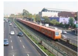
Mexico City - Metro on Grade in Centre of Expressway
