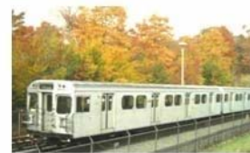
Toronto Metro on Grade
