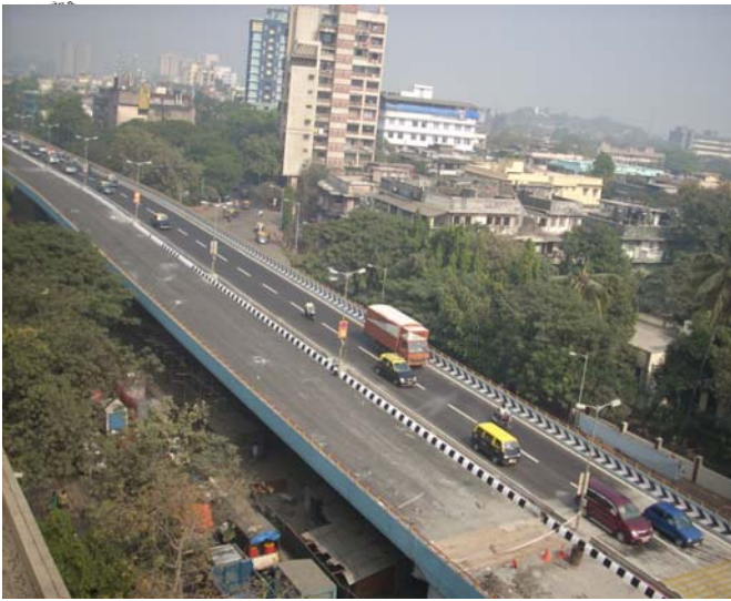
Sion Hospital Flyover
