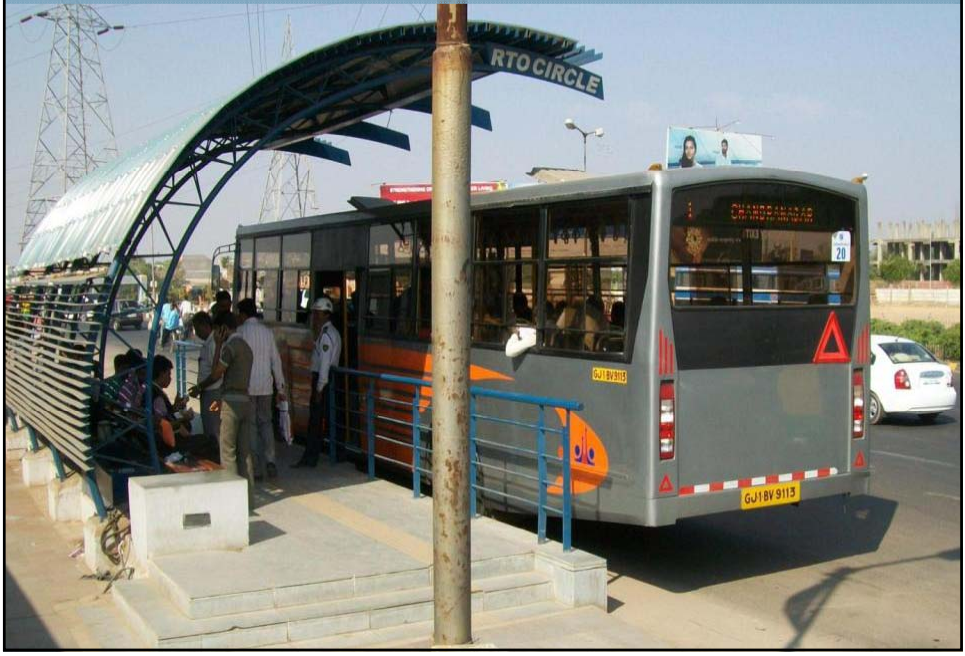
Outside corridor entry from left side door
