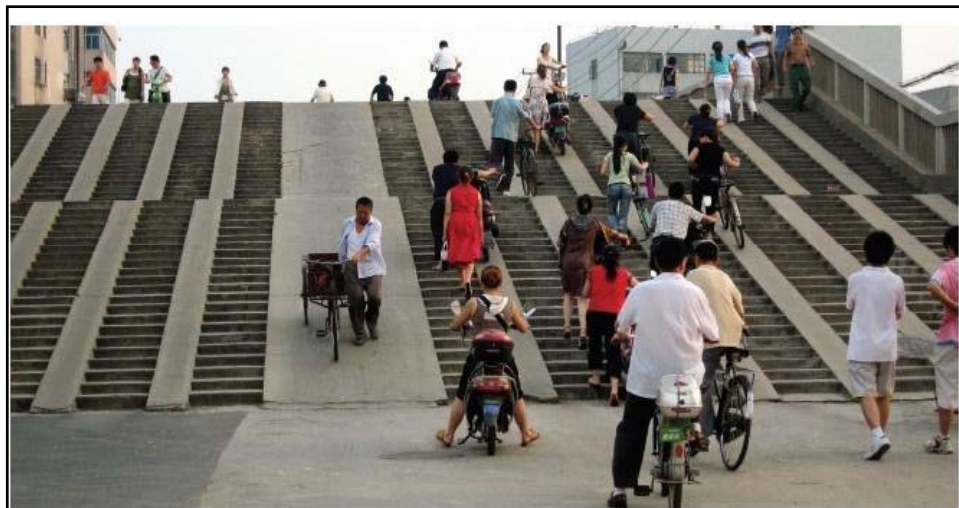
Simple interventions, like adding a ramp to stairs for people using cycles, make crossing more convenient. Changzhou, China.
