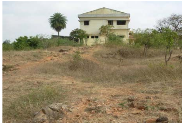
Encroachment at the site
