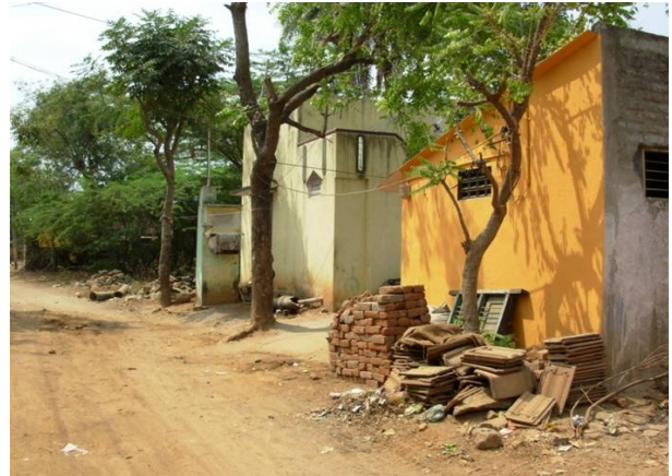
Encroachment at the site
