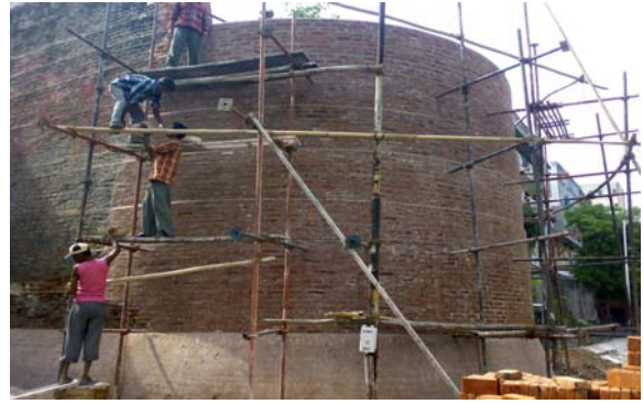
Restoration of Fort Wall (Walled City of Ahmedabad)
