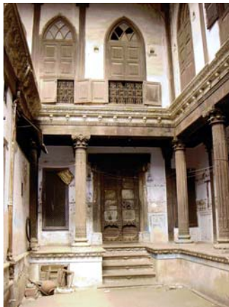
Adaptive Reuse of Traditional Pol Houses
