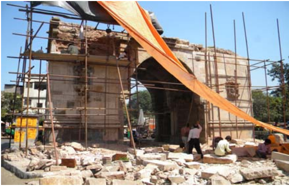
Restoration of Jamalpur Gate (Walled City Gate of Ahmedabad)
