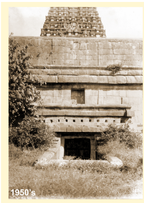
Brihadisvara, Tanjavur – removal of accumulated earth and bringing the original working level back into use
