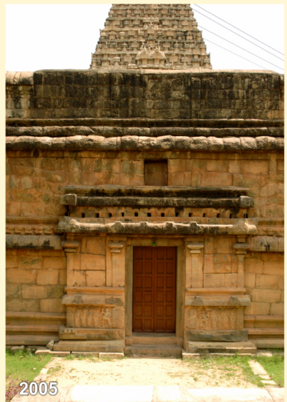
Brihadisvara, Tanjavur – removal of accumulated earth and bringing the original working level back into use
